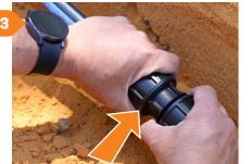
lighten the nut by hand to the point where the nut is touching the flange on the body of the fitting. Do not tighten beyond this point.
