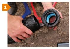
Cut the pipe square, there is no need to chamfer or lubricate the pipe. Then disassemble the fitting.
