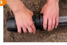
While holding the body tighten the nut all the way to the flange using multi-grips. The fitting is now fully installed.
